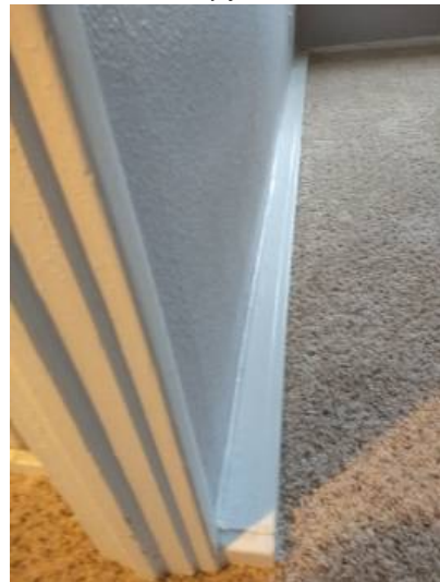
Build out for condensate drain line
