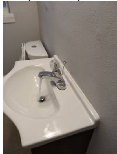
Sink drain plug inoperable
