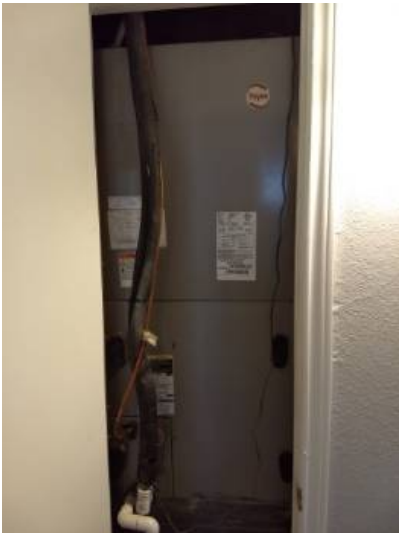
Furnace unit does not have enough clearance to remove.
