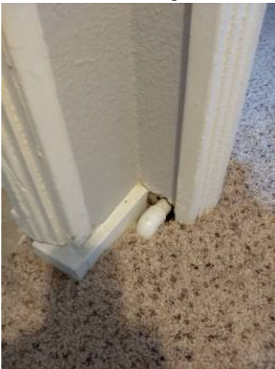
Condensate drain from HVAC runs through hallway
