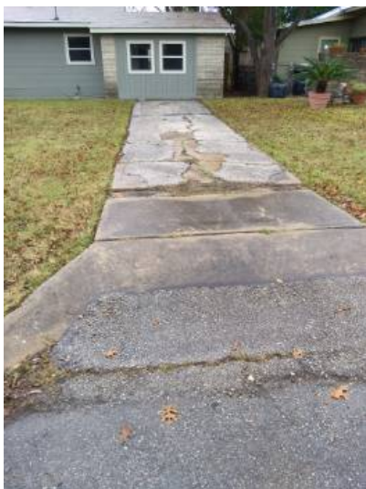
Driveway surface cracked and uneven
