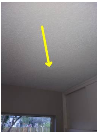
Drywall crack and sagging in bedroom
