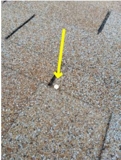
exposed nail in roofing should be caulked
