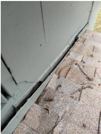
Flashing separating from wall
