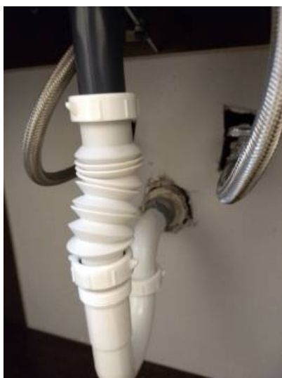
Improper trap and drain connection at vanity
