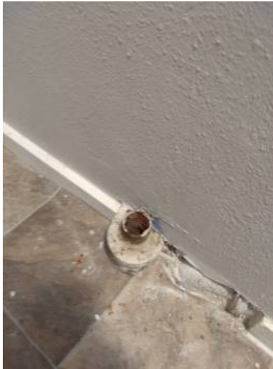
Washer drain at improper height
