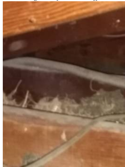
Evidence of pests in attic
