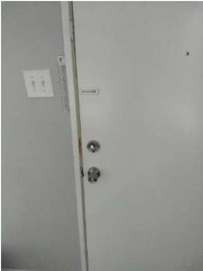
Front door deadbolt operates but does not seat in strike plate.
