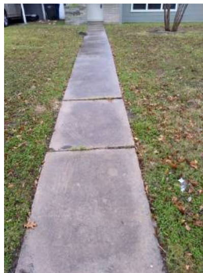
Sidewalk cracked and uneven
