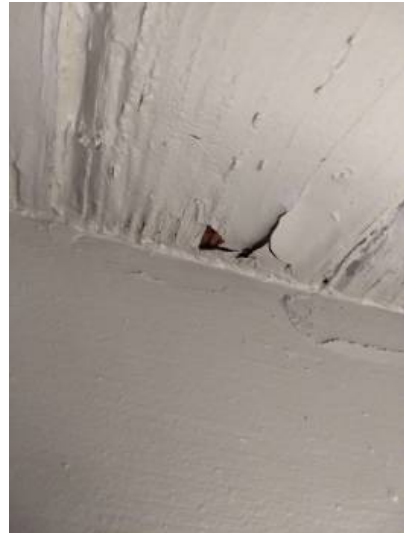
Slight rot found at soffit
