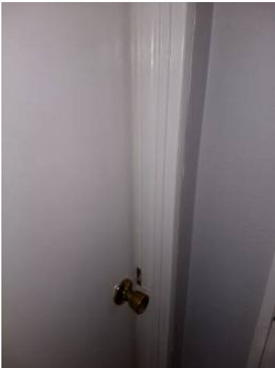
Front door deadbolt operates but does not seat in strike plate.
