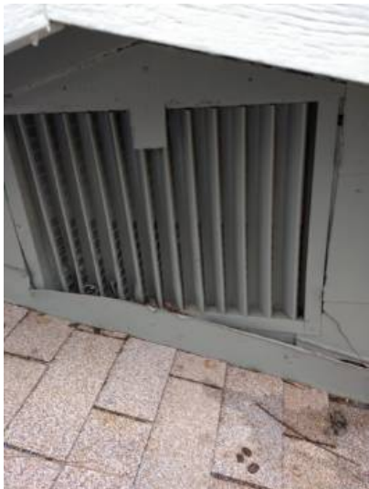
Gable vent installed improperly
