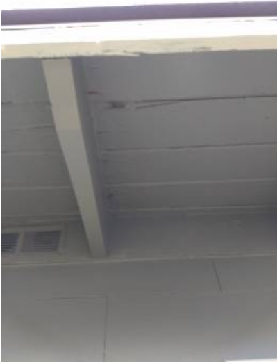
Minor rot to roof decking at eave
