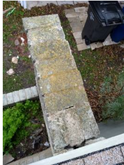
Exposed wall should be properly covered to avoid water infiltration into house
