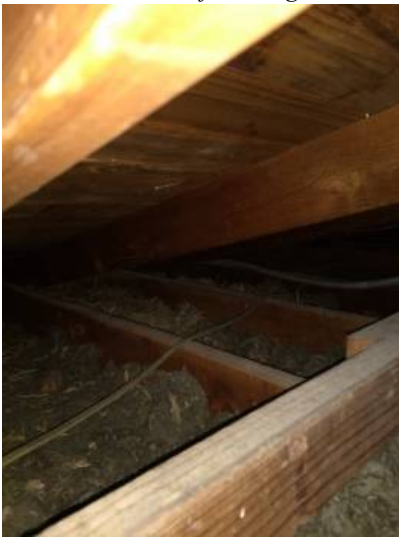
Very low level of insulation in attic
