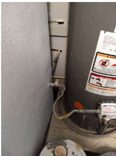
Water heater gas supply was shut off
