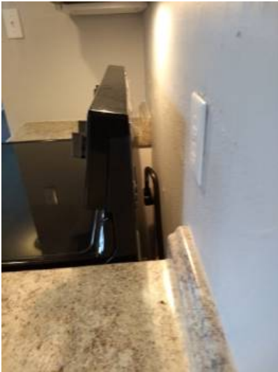
No anti tip device on range.
