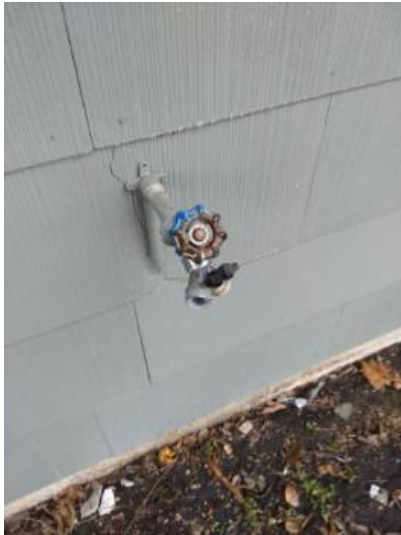
Cannot remove wye from hose bib.
