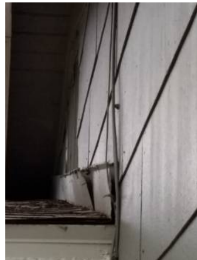
Flashing separating from house at roof junction
