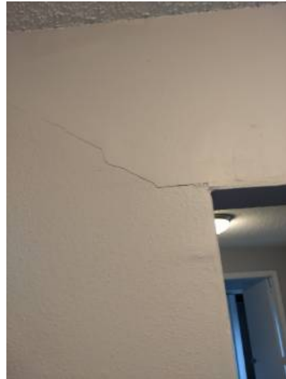
Settlement cracking at door openings
