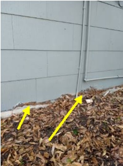
Damage to exterior siding at foundation
