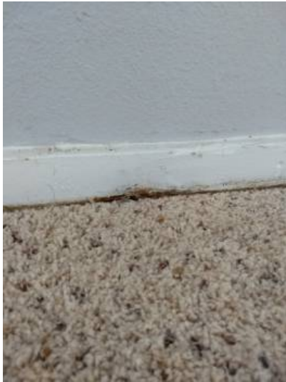
Rot at baseboard in converted garage.
