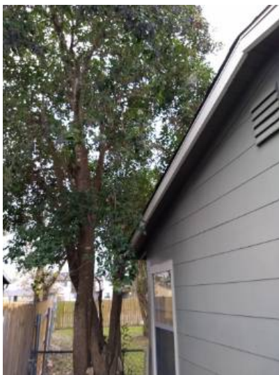
Vegetation contact with roof
